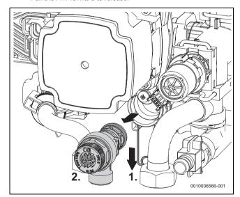
Fig. 97 PRV removal
