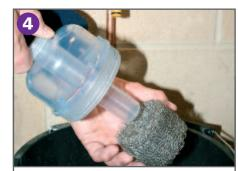
Remove the wire gauze and rinse. Wipe and clean out the clear base. Replace the wire gauze and the magnet cap.
