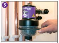
Re-attach the clear base to the top section of MagnaClean TwinTech and tighten until sealed. Do not over tighten.
