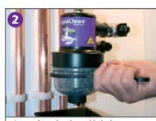
Loosen the canister base with the large spanner while holding the tray beneath. Carefully unscrew the clear base. Allow water to collect in the servicing tray supplied.
