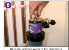
position and vent through the Pro-Fill air vent.
