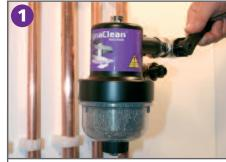
Important - Before commencing any servicing work, turn off the electrical supply to the boiler. Turn both isolation valves to the marked OFF position.
