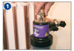
With a standard radiator key, remove the Pro-Fill air vent. The built-in, one-way valve will prevent water from escaping. Attach the chemical adapter and feed in the chemical.
