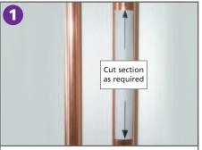
Drain the central heating system or plug-off feed and expansion tank and release the system pressure. Measure and mark an appropriate section when making the connections with elbows as shown (Refer to the Installation Instructions inside the box). When installing above a boiler or other object allow 95mm clearance between the magnet cap to the top of the boiler or other object for the removal of the clear base when servicing.
