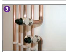
Prepare the pipe and fittings accordingly. Lubricate the olives and assemble the valves on the pipe. Hand tighten.
