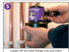
the rubber washers provided. Tighten the flange nuts. Do not over tighten. Refill the heating system.
