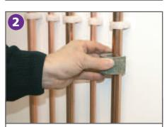
Using a suitable cutter, carefully remove the marked section of pipework to create the correct opening.
