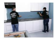
4. ALWAYS dry fit the panels and check the fit.
