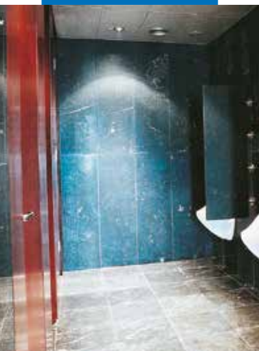
An example of the installation of marble to walls with Keraquick S1 - Feuchtwangen casinò bathroom (Germany)
