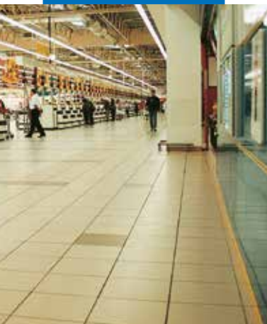
An example of an installation with Keraquick S1 in an Auchan supermarket - Sosnowiec (Poland)
