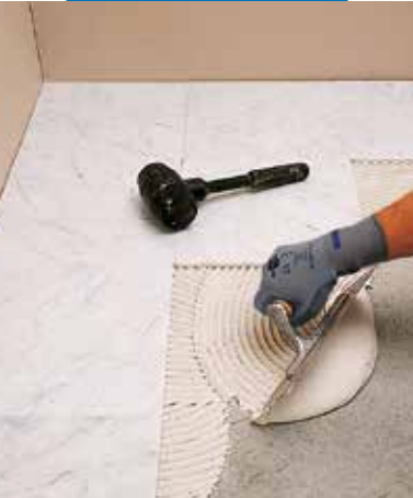
Setting white Carrara marble with Keraquick S1 white
