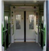
Railway carriage Interior components
